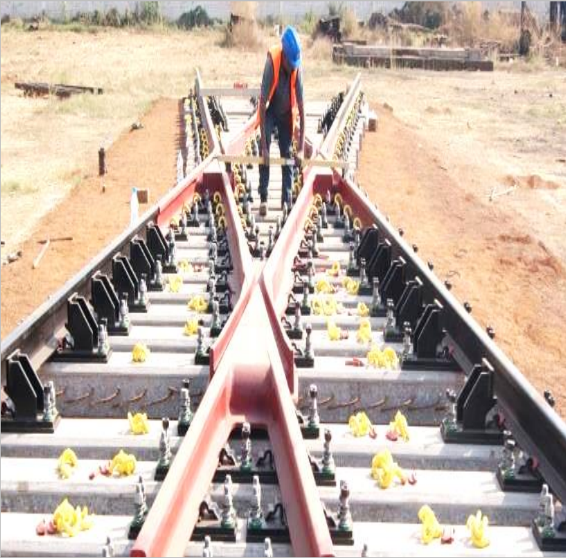
/ Welded CMS Crossings assembly
